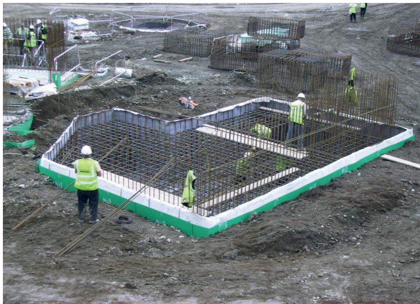
Large Pile Cap combining Corriform and Fosroc Proofex Hydromat System
