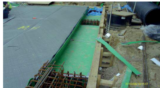
Fosroc Proofex Engage under slab & reinforcement
