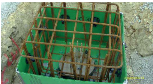
Sealed under slab Pile Head
