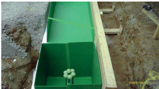
Formwork to slab edge beam
