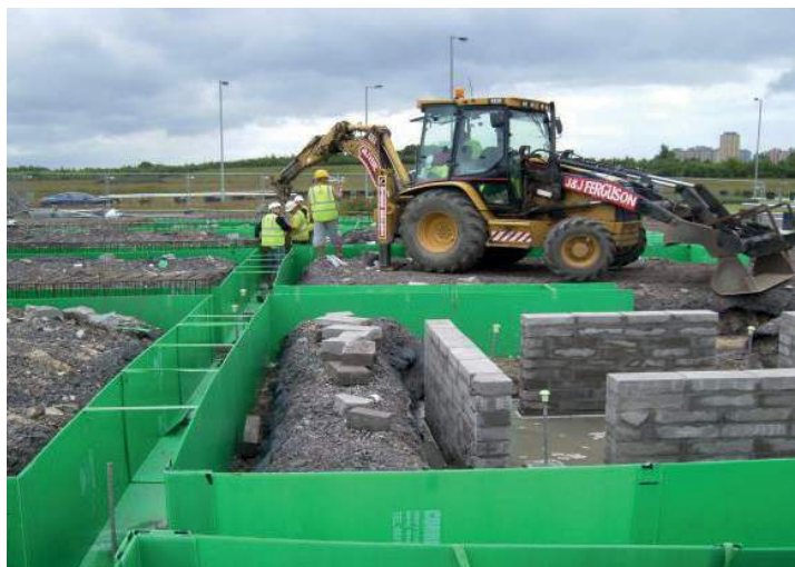
Methane Proofing – On site photo example
