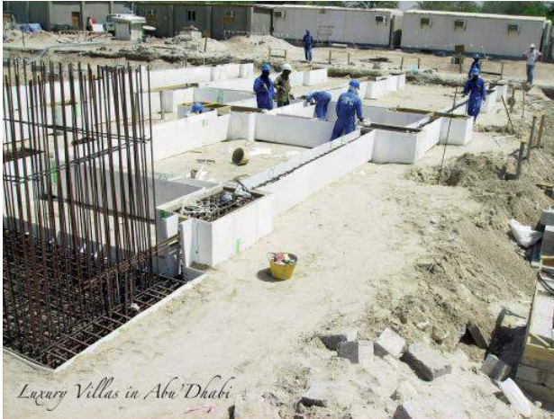
Sulphate contamination proofing
